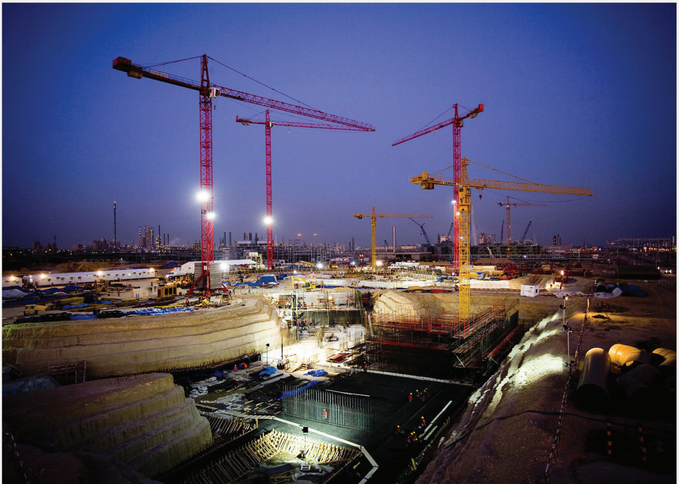
Construction at Shuaiba refinery, Kuwait (Source: 2014, Fluor; Wikimedia Commons)
