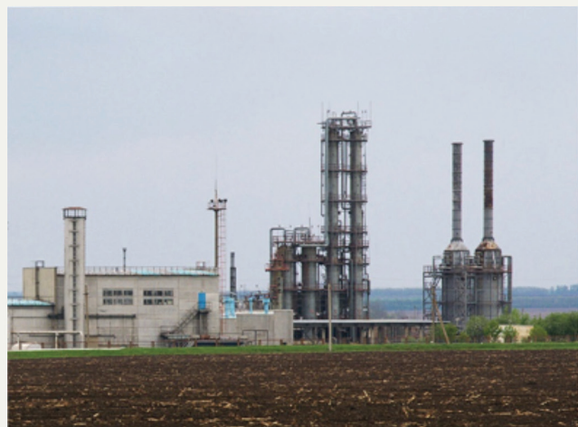
Solohiv gas processing plant, Ukraine (Wikimedia Commons)
